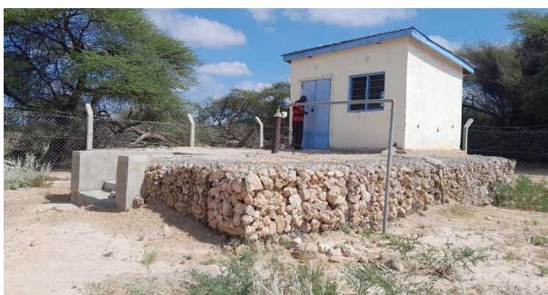
Borehole pump house in Garissa County with borehole operator.
