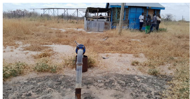
Borehole and pump house with key informant interview in Garissa County.
